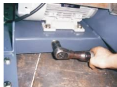
Picture 3-18: Installation of Belt and Belt Pulley 8
