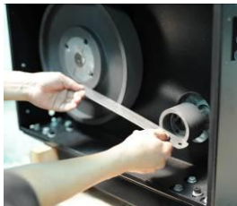
Picture 3-17: Installation of Belt and Belt Pulley 7
