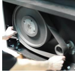
Picture 3-16: Installation of Belt and Belt Pulley 6
