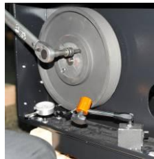
Picture 3-14: Installation of Belt and Belt Pulley 4
