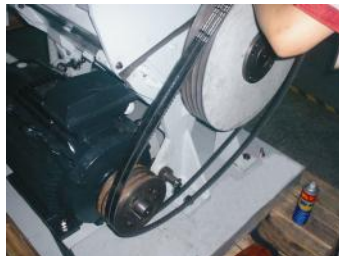
Picture 3-8: Installation of Belt Pulley and Motor 2(SG-3650)
