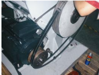
Picture 3-13: Installation of Belt Pulley and Motor 3 (SG-3675)
