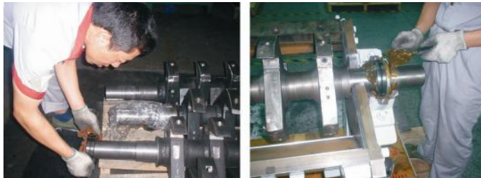
Picture 3-5: Installation of Bearing and Blade Rest
