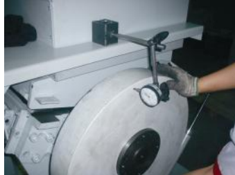
Picture 3-7: Installation of Belt Pulley and Motor 2(SG-3650)
