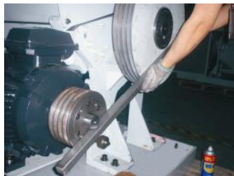
Picture 3-9: Installation of Belt Pulley and Motor 2 (SG-3650)
