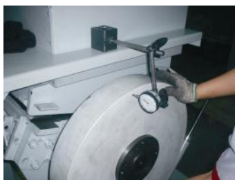
Picture 3-12: Installation of Belt Pulley and Motor 2 (SG-3675)
